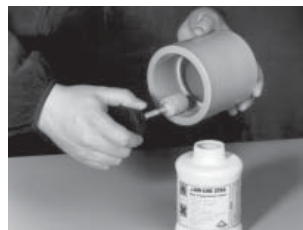
Apply solvent cement to the inside of the fitting
